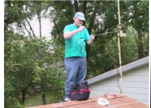
Attaching the other end of the antenna wire.
